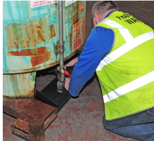
Fitting Dripguard to pallet base
